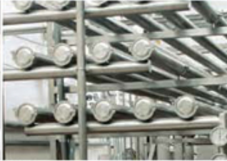
Divo® membrane cleaning
